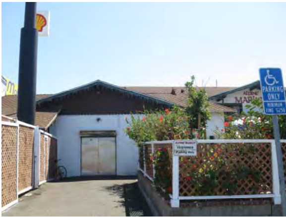
Figure 99. Maintenance area on east end of Alpine Market, looking south.
