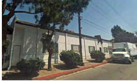
Figure 120. Google street view from 2008 showing windows on south façade.
