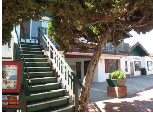
Figure 64. Stairs leading to balcony on north façade of Building 2.
