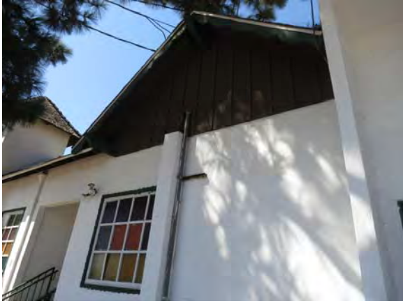
Figure 46. Gable end on east corner of south façade of Building 2.
