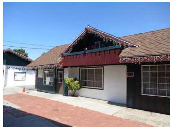
Figure 22. Detail of west gable on south façade of Building 1.
