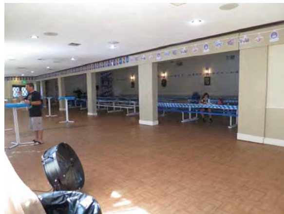
Figure 20. View of interior of Building 1 showing former theater space, looking northwest.
