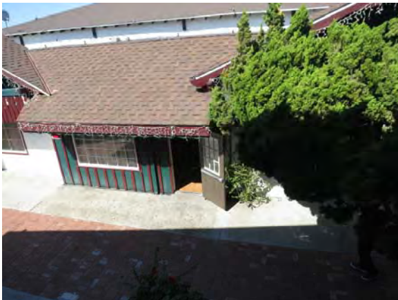
Figure 25. Detail of storefront between gables on south façade of Building 1.
