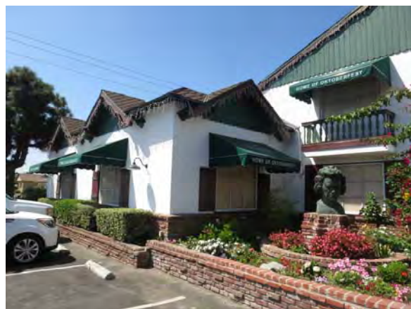
Figure 112. East façade of Alpine Inn looking southwest.
