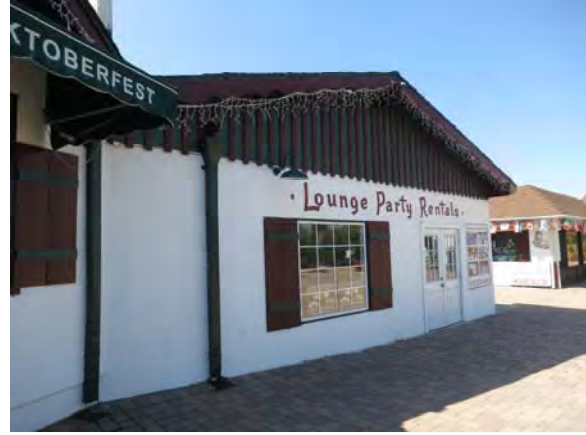
Figure 51. North façade of east wing of Building 2 looking southwest.
