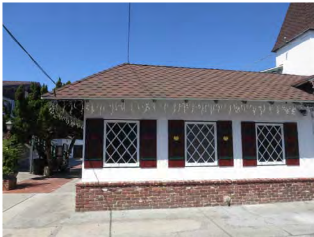
Figure 13. Windows to the south of entrance on east façade of Building 1.
