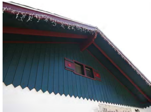
Figure 84. Detail of gable end of Building 4.
