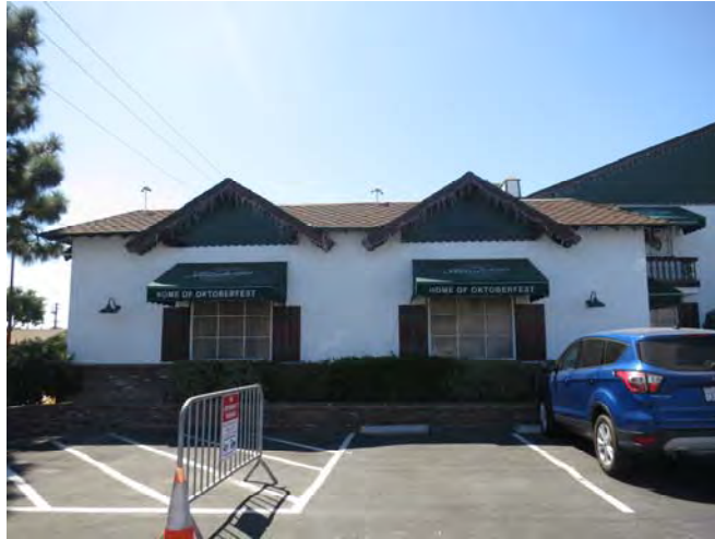
Figure 113. South end of east façade of Alpine Inn looking west.
