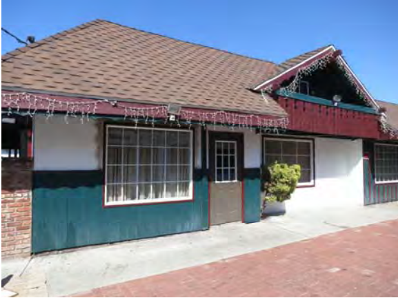
Figure 23. Southwest corner of Building 1 looking northeast.
