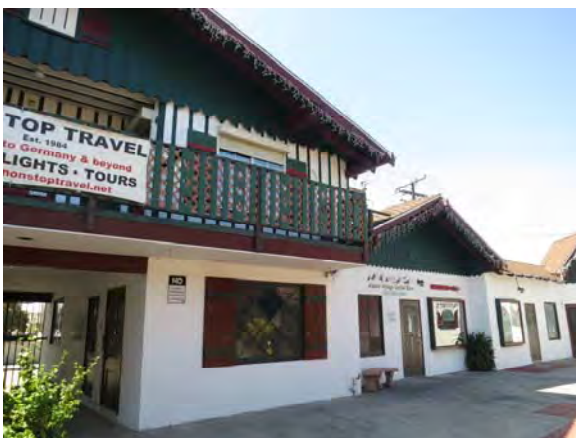
Figure 67. West end of gable on north façade of Building 2.
