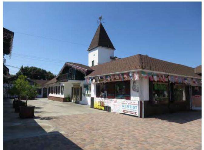
Figure 14. Oblique view of Building 1 looking southwest.
