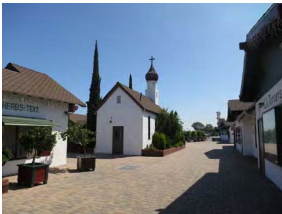
Figure 93. West façade of Chapel looking northeast.
