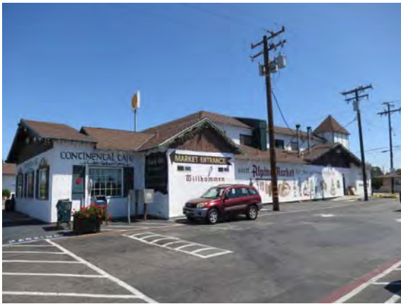
Figure 104. Oblique view of Alpine Market looking southeast.
