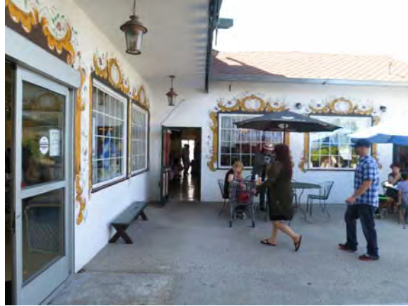
Figure 103. Door at southeast corner of café looking west.
