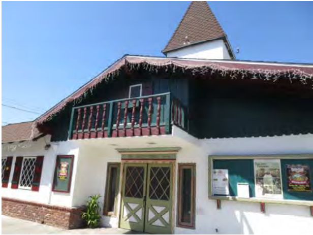
Figure 11. Detail of central balcony on east façade of Building 1.
