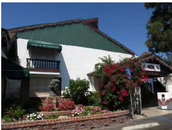
Figure 111. East façade of Alpine Inn looking northwest.
