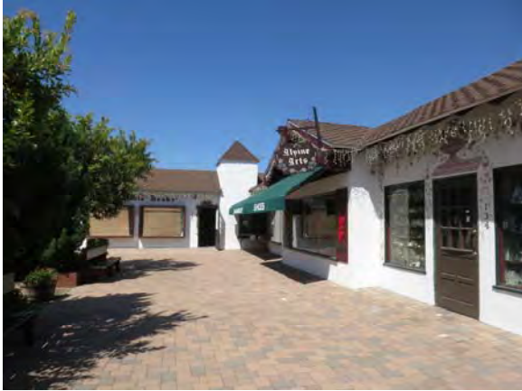
Figure 73. View of Building 3 looking west.
