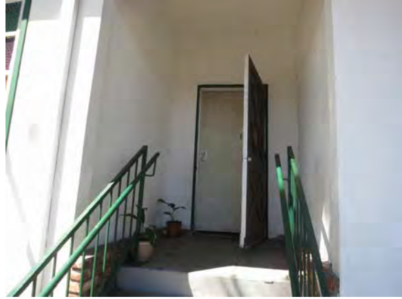
Figure 47. Rear entrance on east end of south façade of Building 2.
