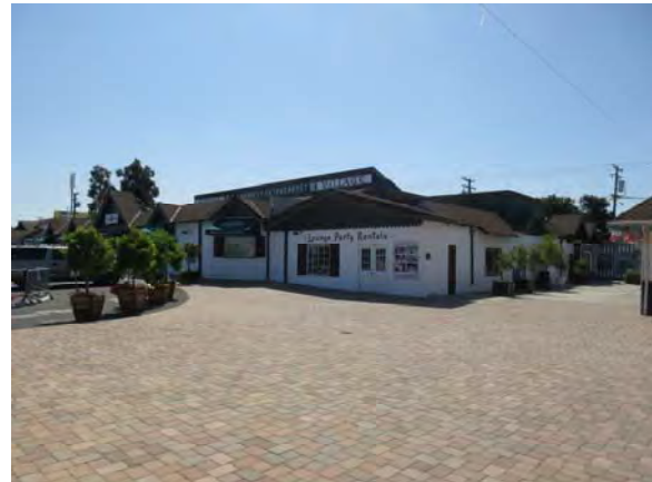
Figure 53. Oblique view showing east wing of Building 2.
