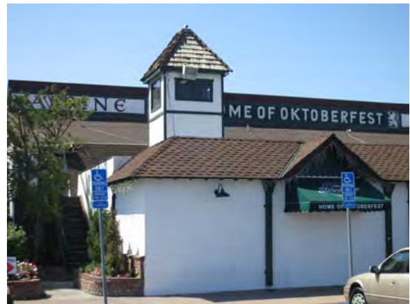
Figure 115. Tower on northeast corner of Alpine Inn.
