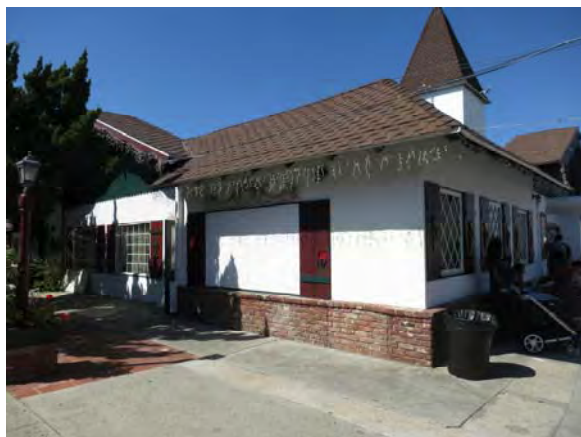
Figure 27. Wall at southeast corner of Building 1.
