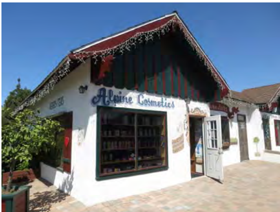
Figure 75. Building 3 southeast corner store looking northwest.
