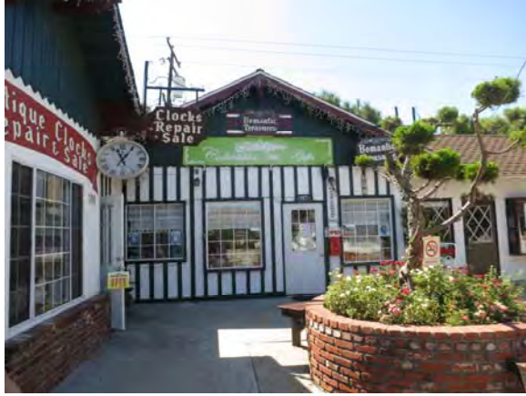
Figure 60. Store at east corner of north façade of Building 2.
