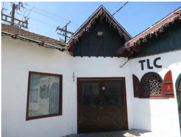
Figure 69. Former entrance to Alpine Inn Restaurant in northwest corner of Building 2.
