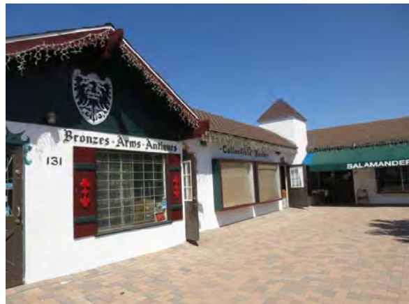
Figure 76. East façade of Building 3 looking northwest.
