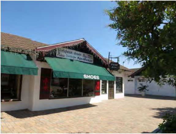
Figure 78. South façade of Building 3 looking northeast.
