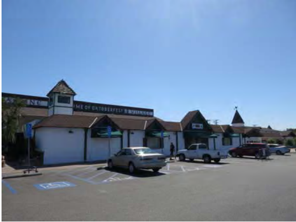
Figure 116. North Façade of Alpine Inn looking southwest.
