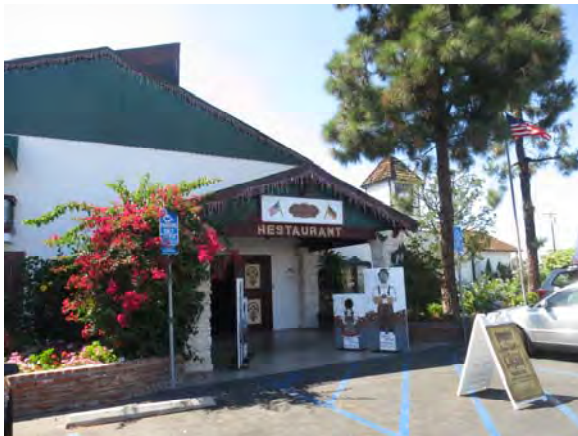
Figure 109. Front entrance on east façade of Alpine Inn Restaurant.
