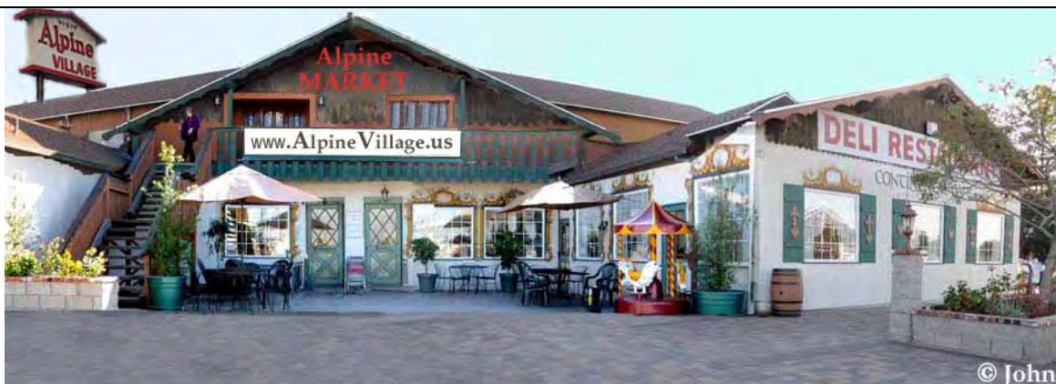
Figure 98. Pre-2008 photo showing original Alpine Market doors.
