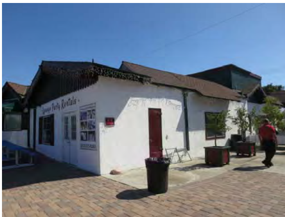
Figure 56. North end of east wing of Building 2.
