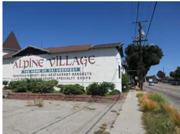
Figure 49. West façade of Building 2 looking east.
