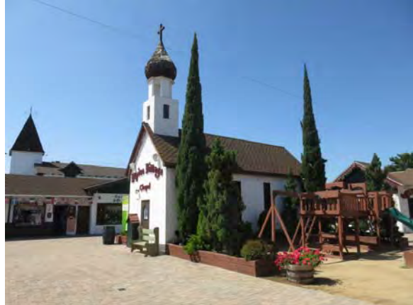
Figure 92. North façade of Chapel looking southwest.
