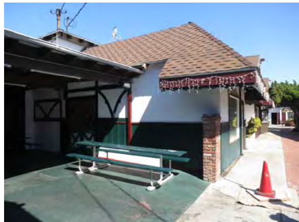
Figure 32. Doors at south end of west façade of Building 1.
