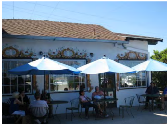
Figure 102. Detail of windows on east façade of café looking west.
