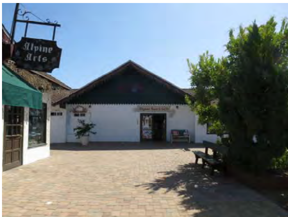
Figure 83. West gable of Building 4 looking east.
