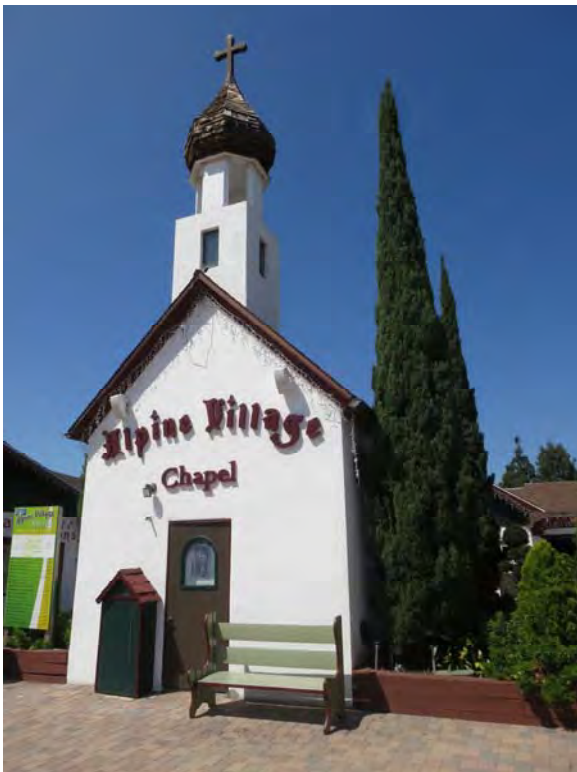
Figure 89. Oblique view of east façade of Chapel.
